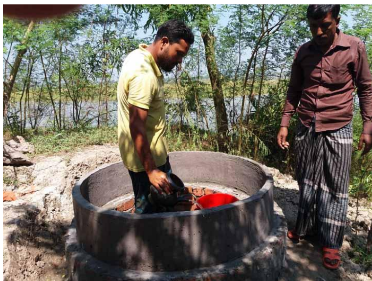
Installation of rain water tanks, Picture-10
