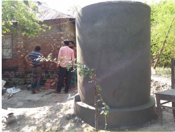
Installation of rain water tanks, Picture-11
