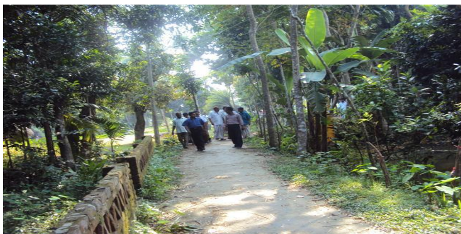
Baro Raghunathpur Drainage Sub-project Area
